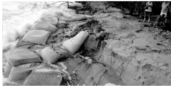
Figure 1: Removal of Top Container by overtopping
